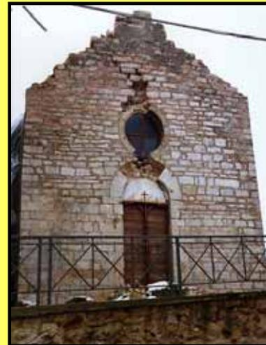
damage in the panels to the sides of the portal and horizontal to the center of the façade
