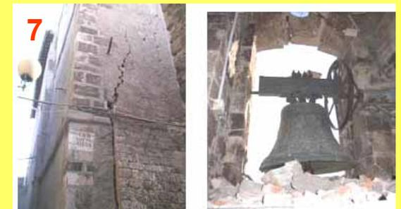
**DAMAGE INDEX**  $I_d = 0,546$  (seismic damage  $I_{mcs}$  7) +  $0,158$  (morphological amplification) =  $0,704$
